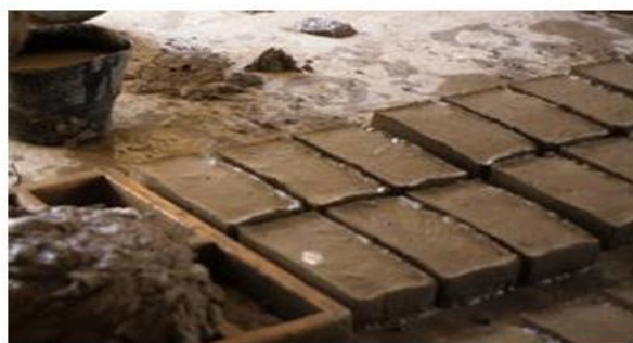
Fig.1.1: Manual brick making
